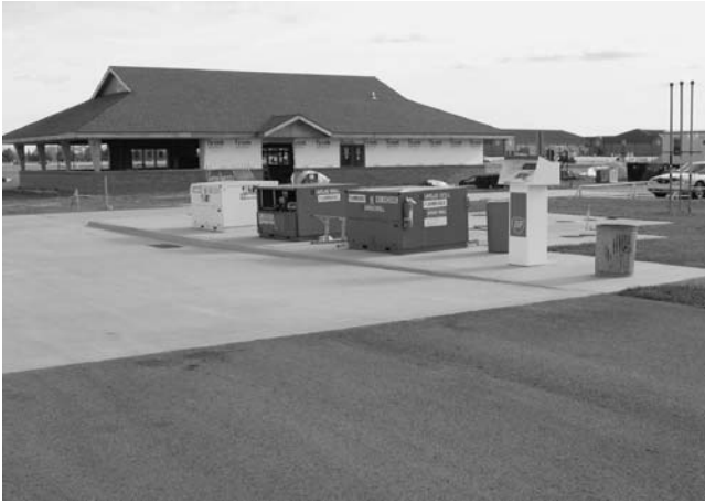
FIGURE 3 Self-fueling facility at a general aviation airport.
