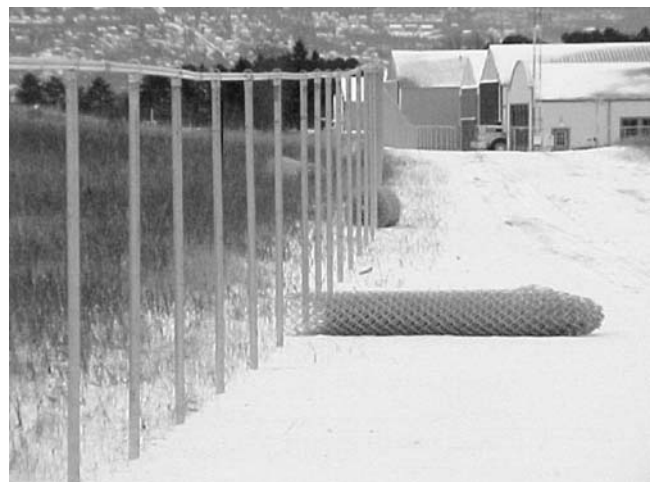
FIGURE 6 New installation of perimeter fencing at a general aviation airport.
